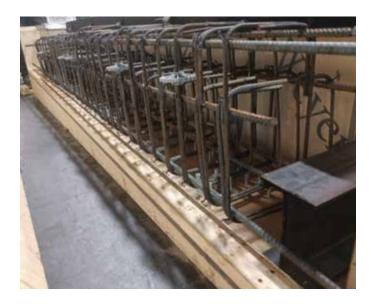
We tackled some interesting products this year. This is a custom sidewalk vault (one of three) with many different critical angles to match the existing sidewalk grade. The 8' x 4' hatch cast in along with bondouts for grates structure was very challenging due to tight spacing for hardware, rebar, and then some concrete!
