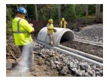
Often, as with the Arch, we use one form for something completely different than what we purchased that form for. In Portland, we used a 38Y Electrical vault (6' x 12') for a large drainage structure. This was the Bedford Street job that we did with Shaw Brothers Construction. This vault has a 60" ADS
